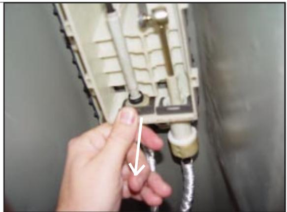
**STEP 8.** Remove knob by pulling up. Excessive force may be required. BE CAREFUL!
